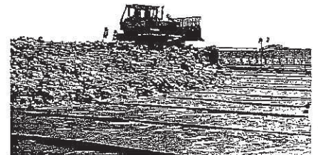
Mirafi® woven geotextile used to filter leachate in a landfill
