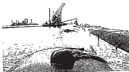
Geotube® containment units used to construct dykes for land reclamation
