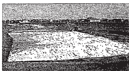
Mirafi® woven geotextile used for basal reinforcement of embankment on soft soil
